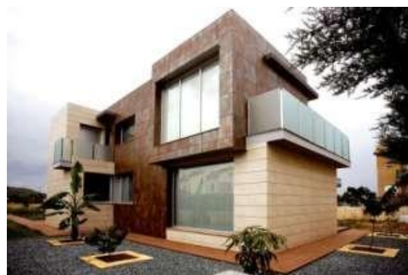
Figure 14: Ceramic and porcelain, cladding tiles for facades, with natural effects
