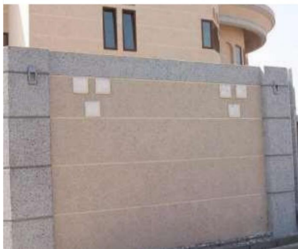
Figure 21: The final form of stone-breaking paint, with durability and resistance of rain and humidity
