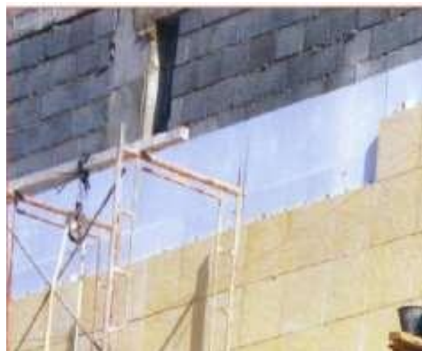
Figure 5: Polystyrene is a thermal and waterproofing insulation
