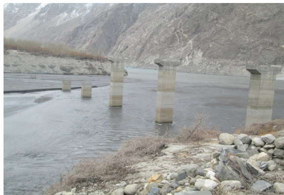
Figure12: New Sheshkat Bridge
