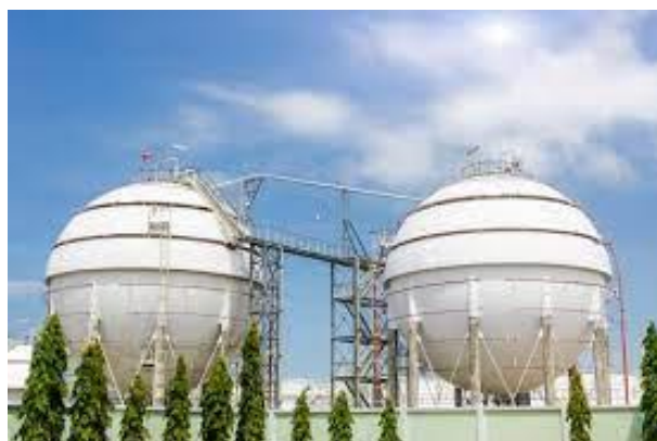
Figure 4: Gas Storage Tanks
