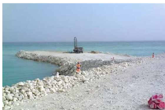
Fig. 4: Prepared ground in the sea for offshore structures location
