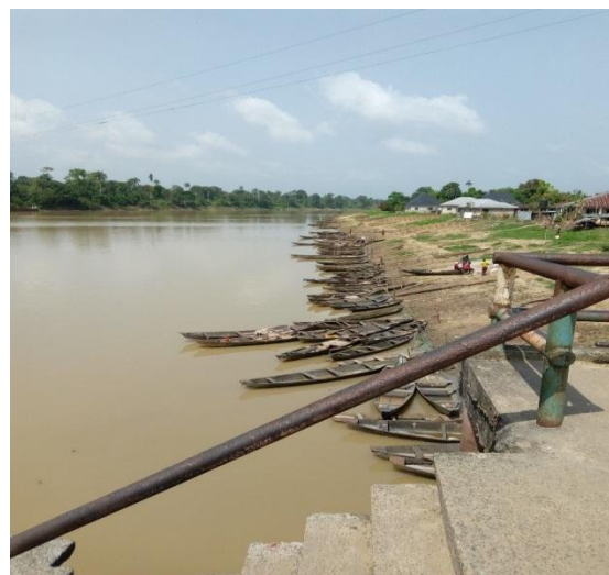
Figure 1: The Polaku jetty front
